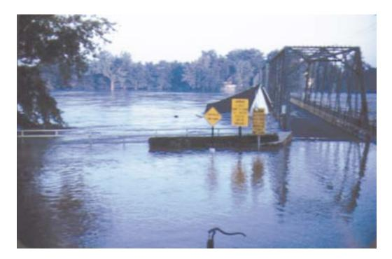
While the Washington Crossing Bridge held, the Yardley Bridge finally gave way to massive pressure exerted on the debris that had piled up against it. It would later be temporarily restored with the wooden trusses of a "Bailey" bridge, but ultimately, it would be replaced with the Scudders Falls span, located in a less vulnerable spot downstream.
